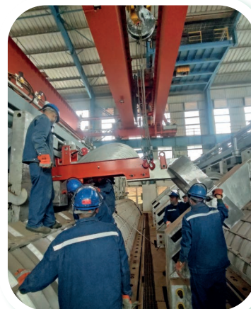
Emergency busbar installation training
